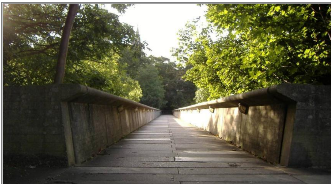
ABOVE: A sunny day at Kingsgate Bridge
