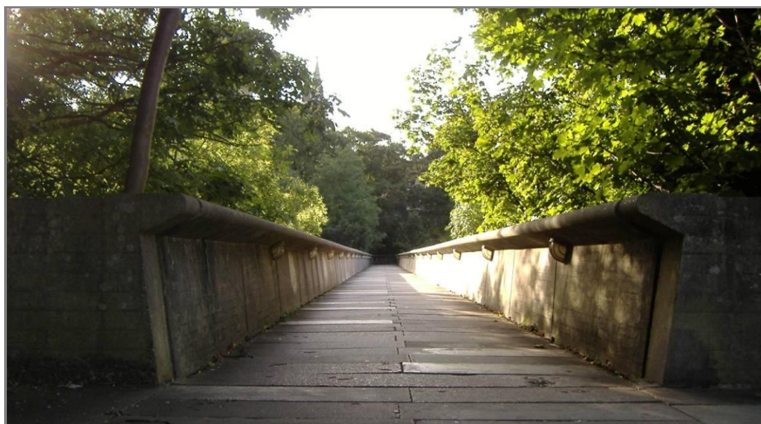
ABOVE: A sunny day at Kingsgate Bridge
